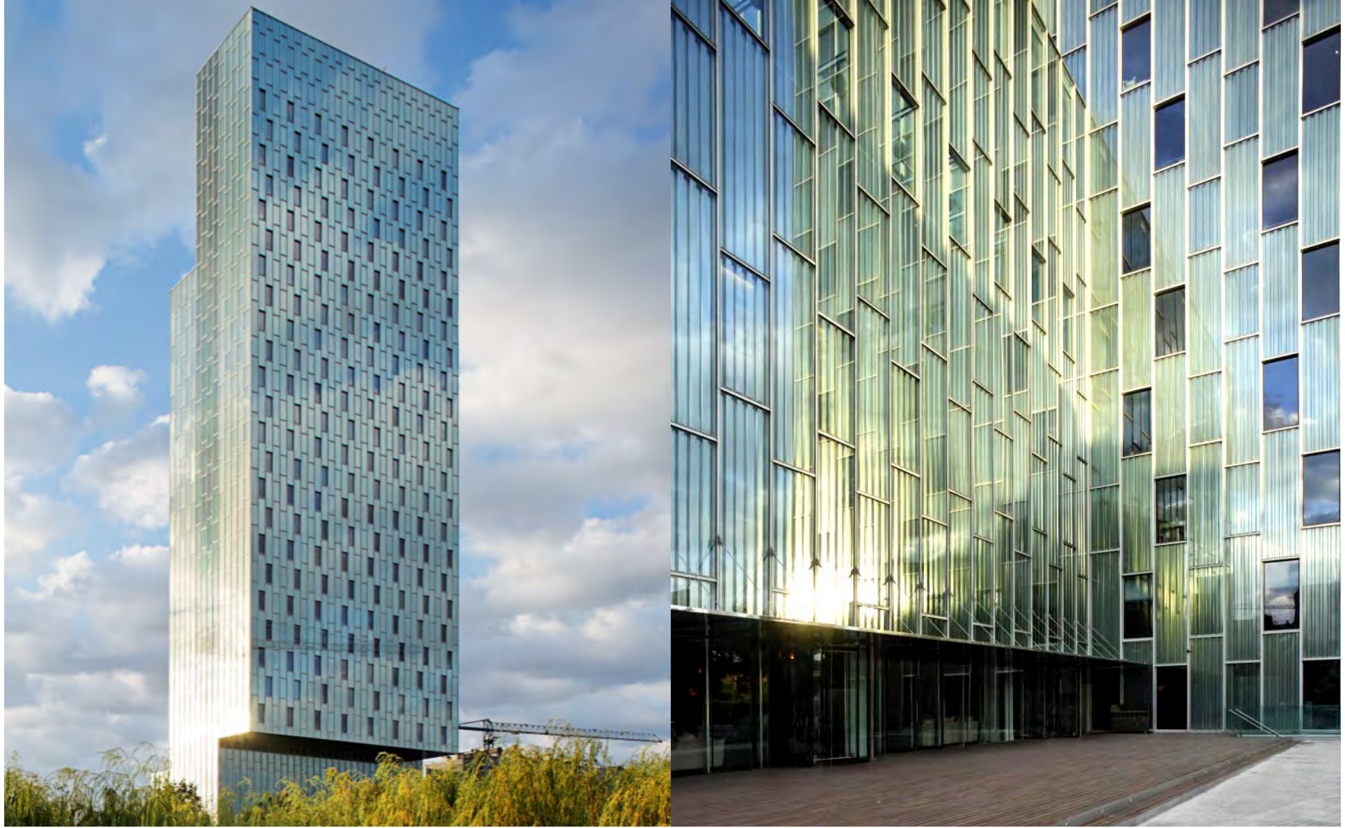
HOTEL ME, Barcelone - Spain / Architect: Dominique Perrault © Dominique Perrault Architecture/ Nuance 316L d'aspect Uginox Bright
